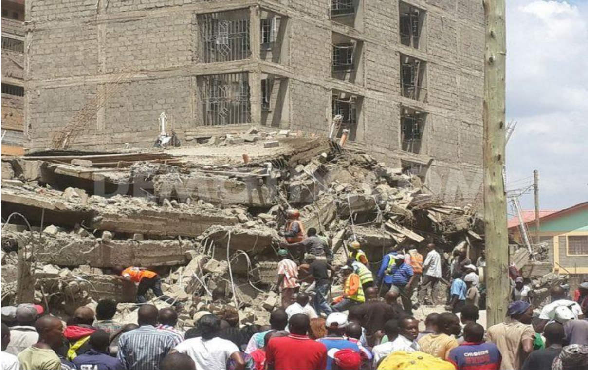
Figure 2: Collapsing buildings in Nairobi (the-star.co.ke, 2015)
