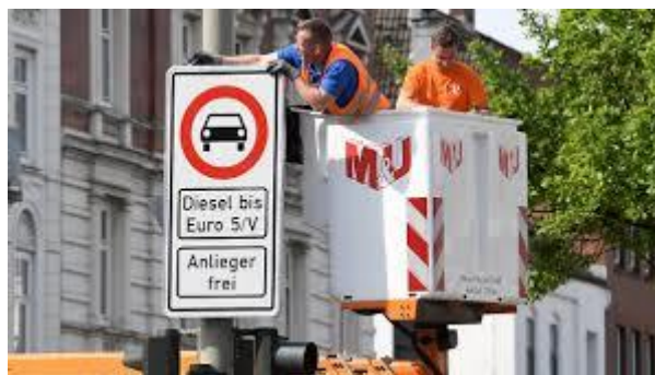
Roadmen setting up signs for diesel driving bans in the city of Hamburg
