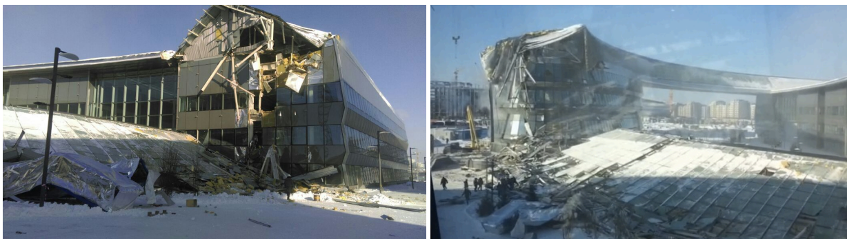
Figure 4. The photos of the demolished structures on the EXPO-2017 site
