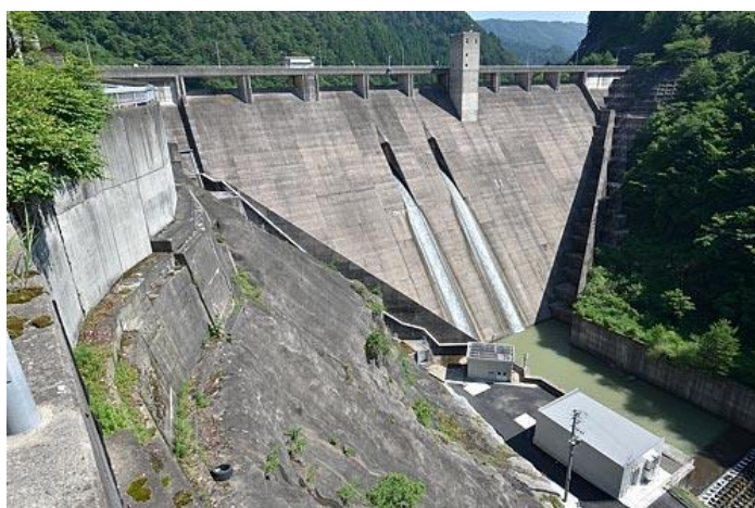
Figure 5: Atagi SHP using the existing dam facility
