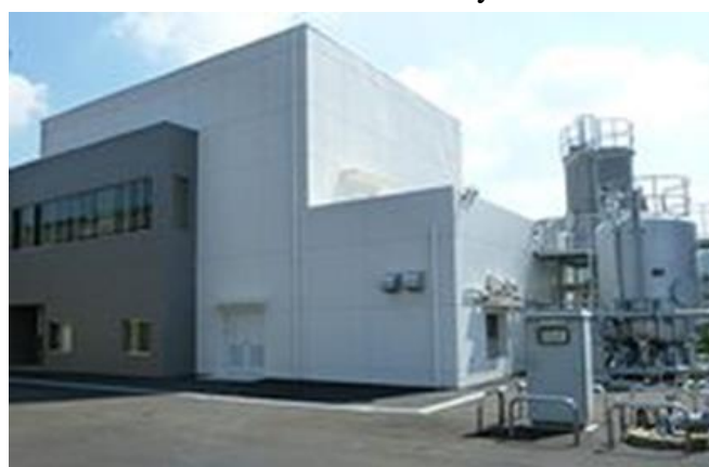
Figure 7: Ikoma Yamazaki Water Purification Facility
