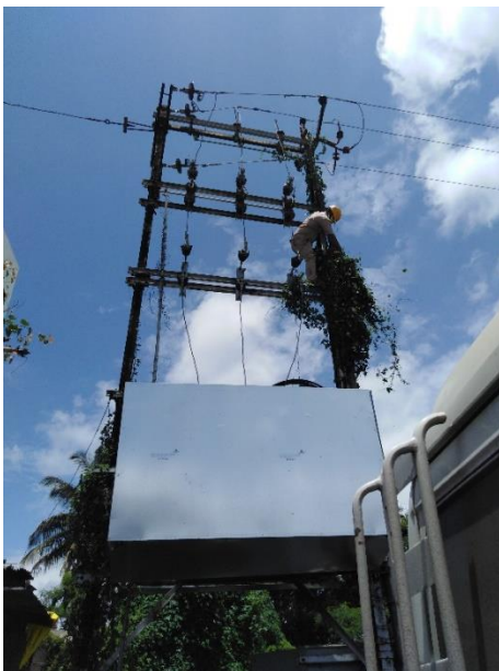
Figure 2: Wireman doing preventive maintenance work
