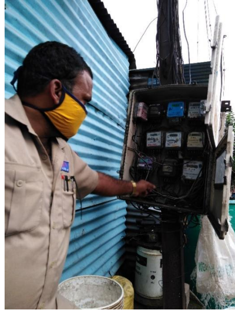
Figure 5: Wireman checking meter reading for consumer complaint
