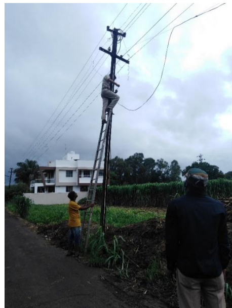
Figure 3: Wiremen changing the service wire on connection
