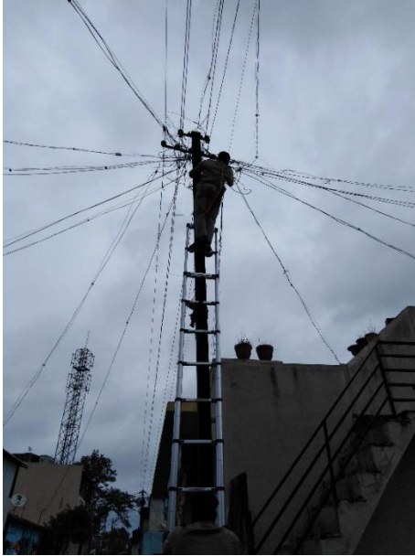
Figure 4: Wireman checking the carbon at the wire connection
